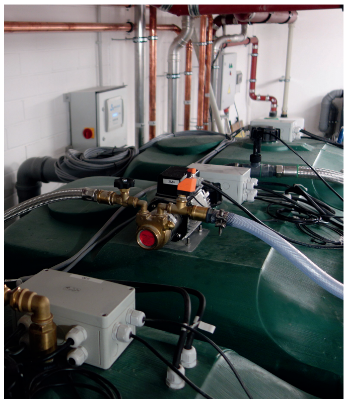
Figure 5: PowerClear MC 5000 gray water system with three tanks at a capacity of 3,000 liters each for installation in buildings. Capacity: Five thousand litres of service water supplied daily.
