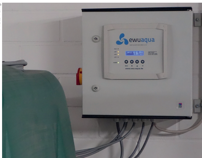
Figure 4: PowerClear MC 5000 gray water system with fully automatic control, potential-free contact integrating alarm signals into the building's services.
