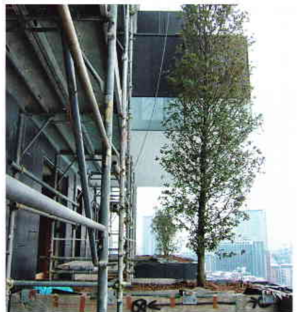
Plant tub as balcony balustrade on the 14th floor being planted in February 2013. Shrubs and ground-cover plants will also be planted. © König
